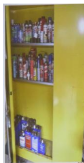
Illustration 4: Storage cabinet for flammables
