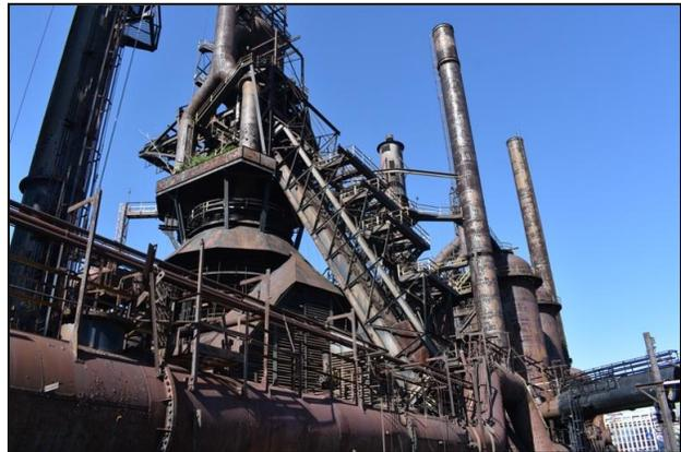
Photo 7: Skip Loader for Blast Furnace
